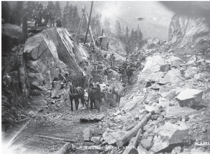
YA #5266 / Caption: Midnight on the grade. [View of a group of W.P.&Y.R. labourers busy at work with pick axes, sledge hammers and shovels clearing the grade of boulders. A team of horses in the foreground and a jerry-rigged hoist in the background are used to remove the larger obstacles.]
